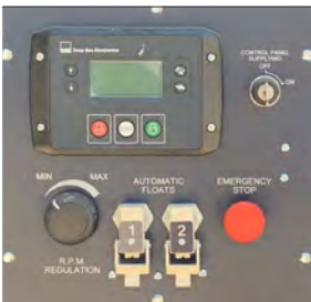
Level Control System - Plug ins for float controls
