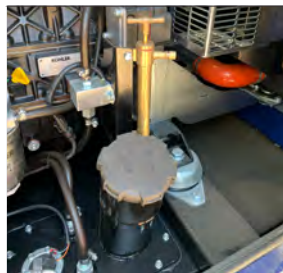
Engine Drain Pump To avoid oil spills during servicing
